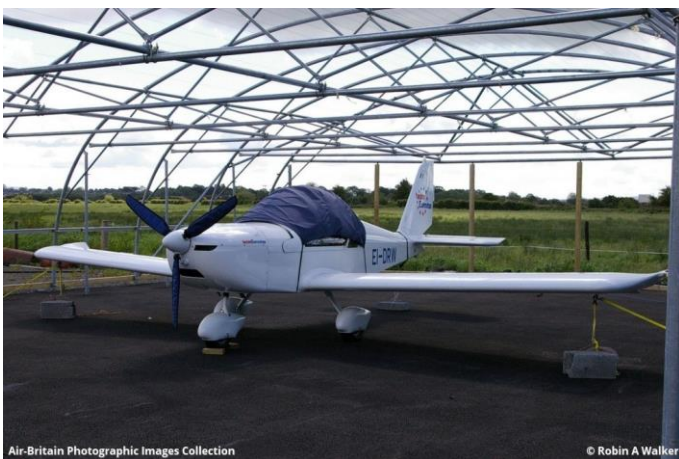
Coonagh based EI-DRW Eurostar in the second club hangar before the roof went on!
